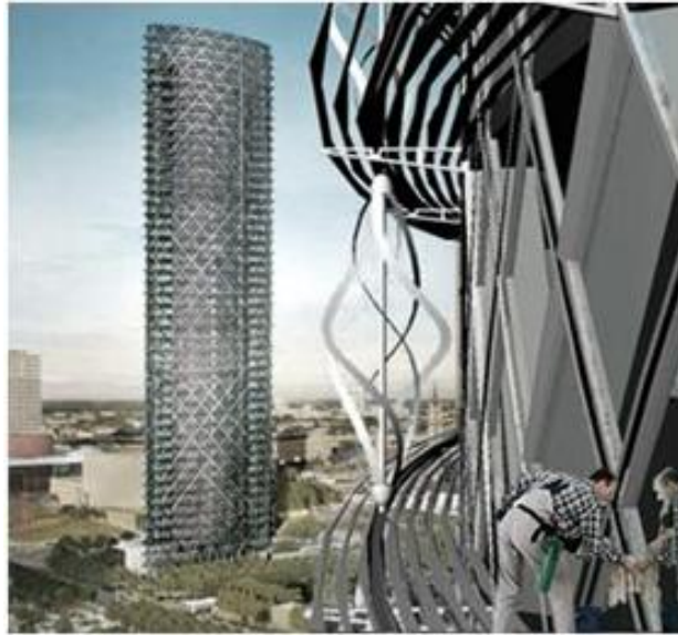
Figure 10: Concept illustrating integration of VAWT's in a streamlined building
